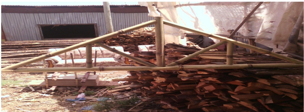
Bamboo roof truss
