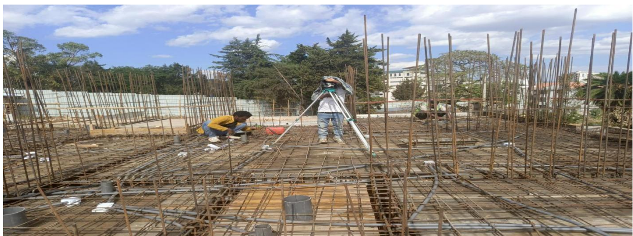
Figure 4. 15: Floor Leveling Check before concrete casting
