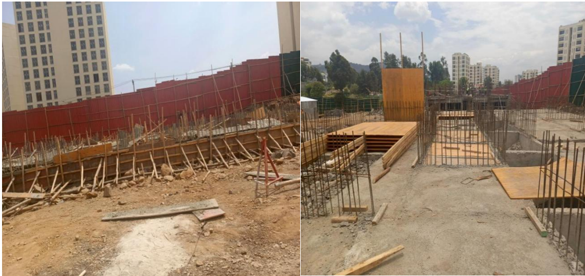
Figure 4. 6: Grade Beam form-work and Concrete work of Ginfile project
