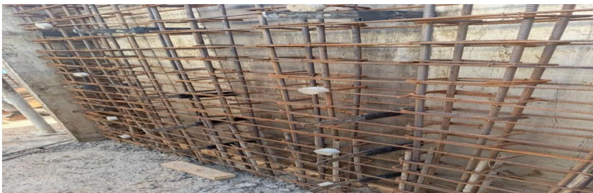
Figure 4. 7: Erection of Vertical and Horizontal Reinforcement bar
