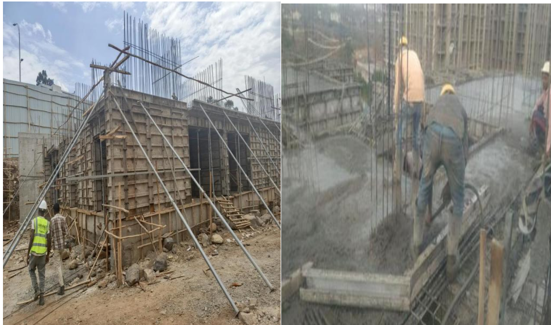
Figure 4. 16: Monolithic slab, beam and wall concrete casting process
