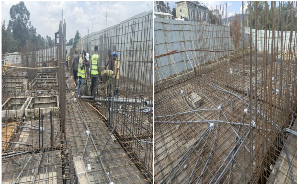
ure 4. 14: Slab reinforcement bar and Electrical Conduit installation
