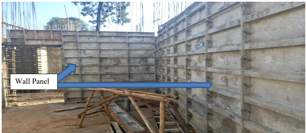
Figure 4. 10: Wall Panel installation and Middle beam erection
