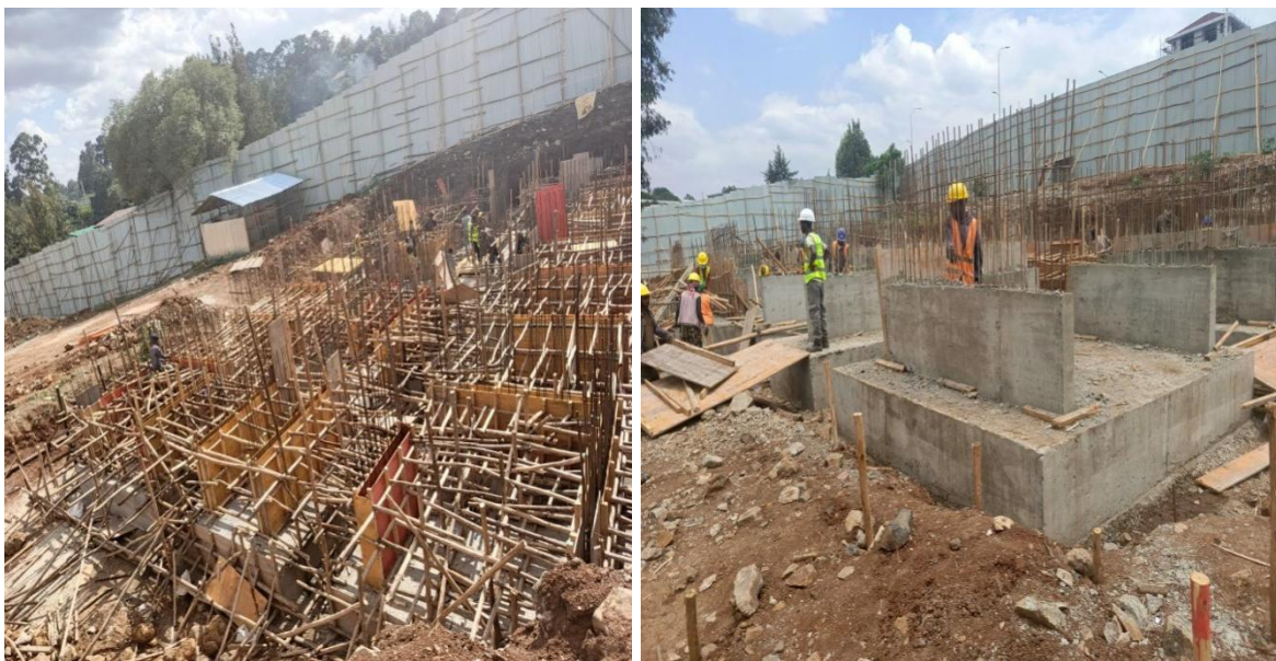
Figure 4. 5: Foundation Column form-work and Concrete work of Ginfile project
