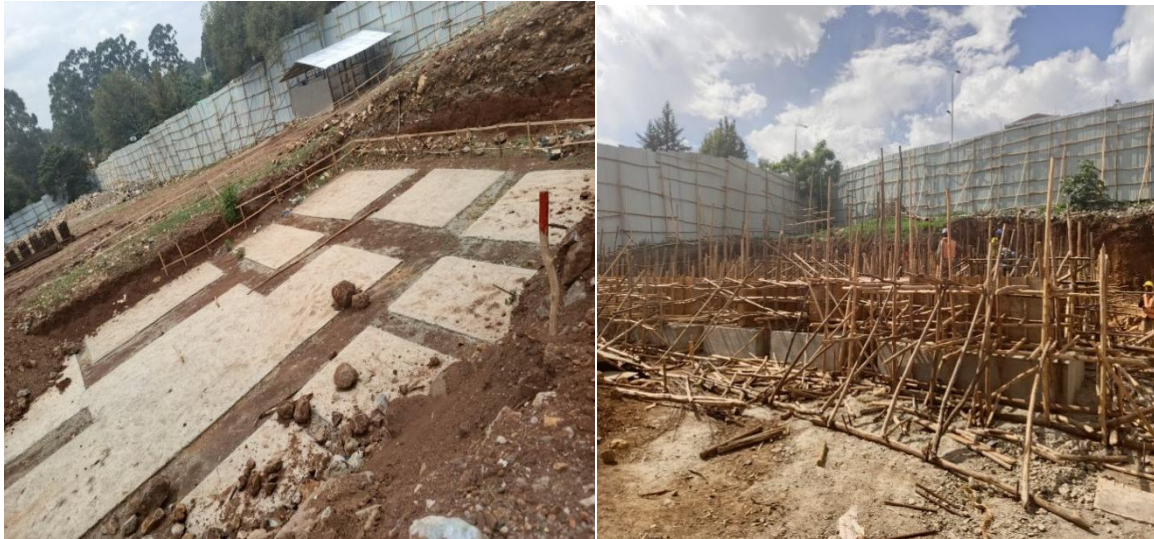
Figure 4. 4: Lean concrete preparation and footing pad concrete work of Ginfile project
