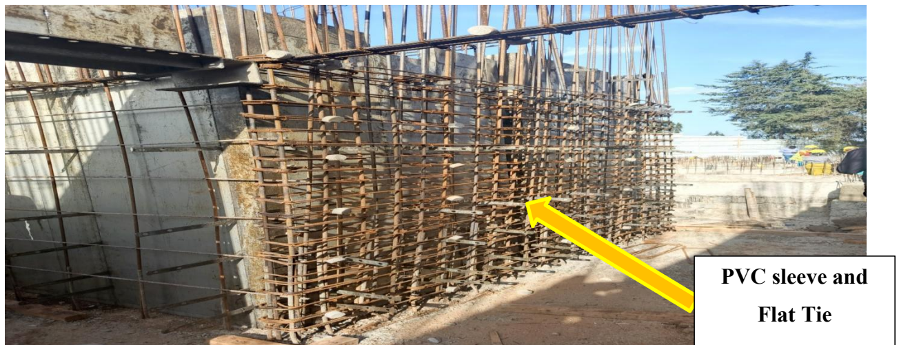
Figure 4. 9: PVC Sleeve and Flat tie installation
