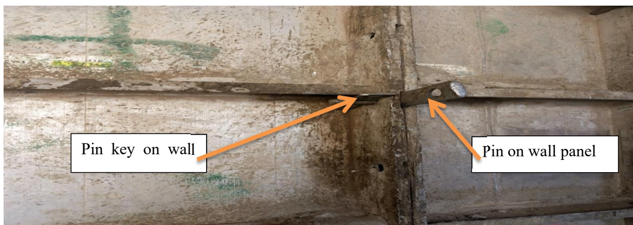
Figure 4. 11: Wall panel pin and pin key
