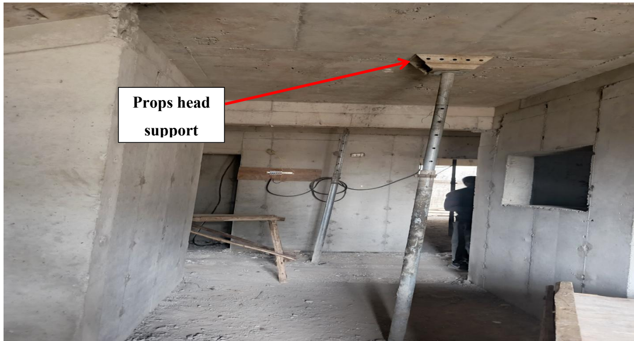
Figure 4. 19: Props head support after de-shuttering
