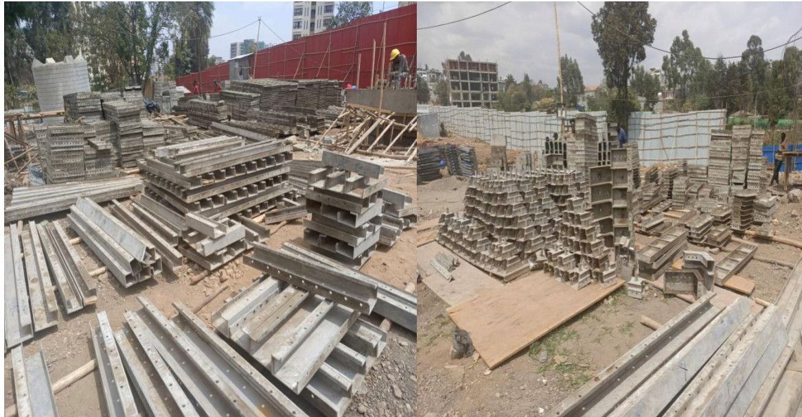
Figure 4 3: Kumkang Aluminum form-work Component material Stock on site Ginfile project
