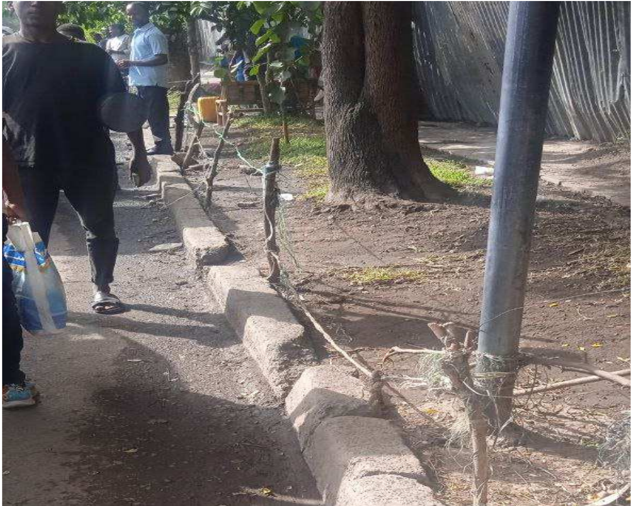
Figure 0-1.1 Road with no walkway people forced to share the road with the cars
