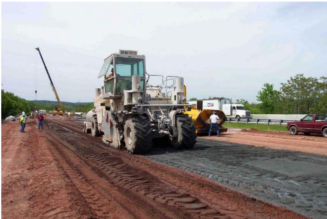
Figure 2. 3 Showing Fly ash soil stabilization in road construction.
