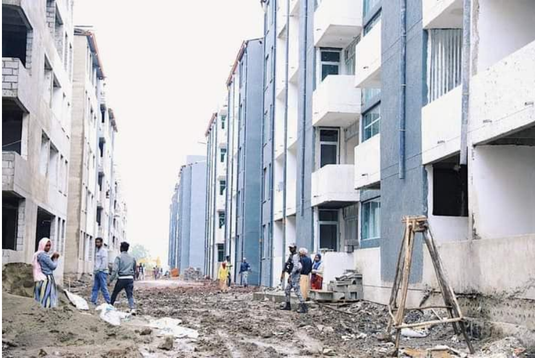
Figure 6 ECWC's 5000 Homes Project Using Precast Frames
