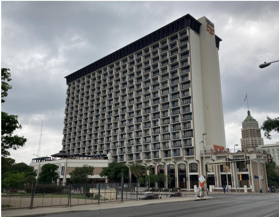
Figure 5 Hilton Palacio Del Rio Hotel constructed by precast
