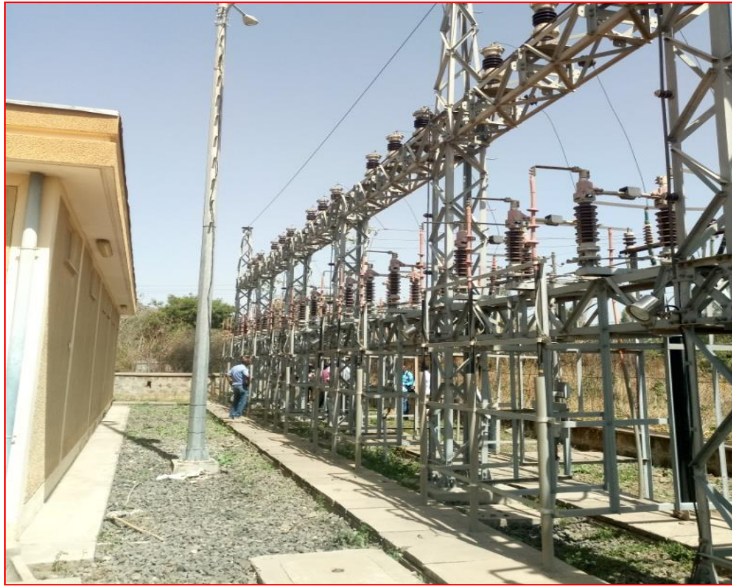
Figure 4.6: Seven outgoing feeders L1 to L7 (gantry)
