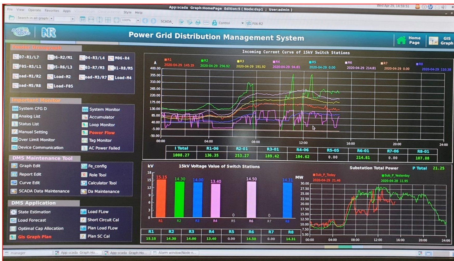
Figure 4.17: Home page of SCADA Power Grid Distribution Management System
