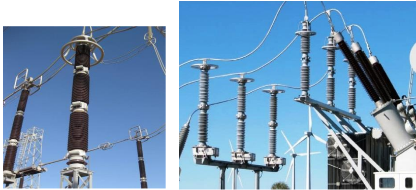
Figure 4.13: Lightning arrester [33]
