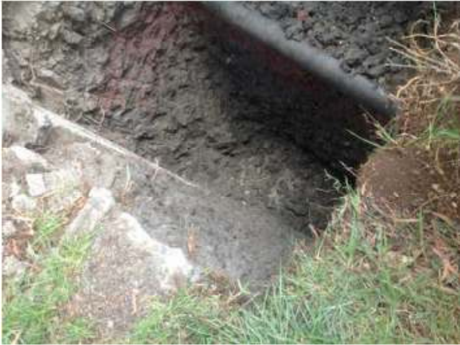
Figure 9. No selected material is found around the footing
