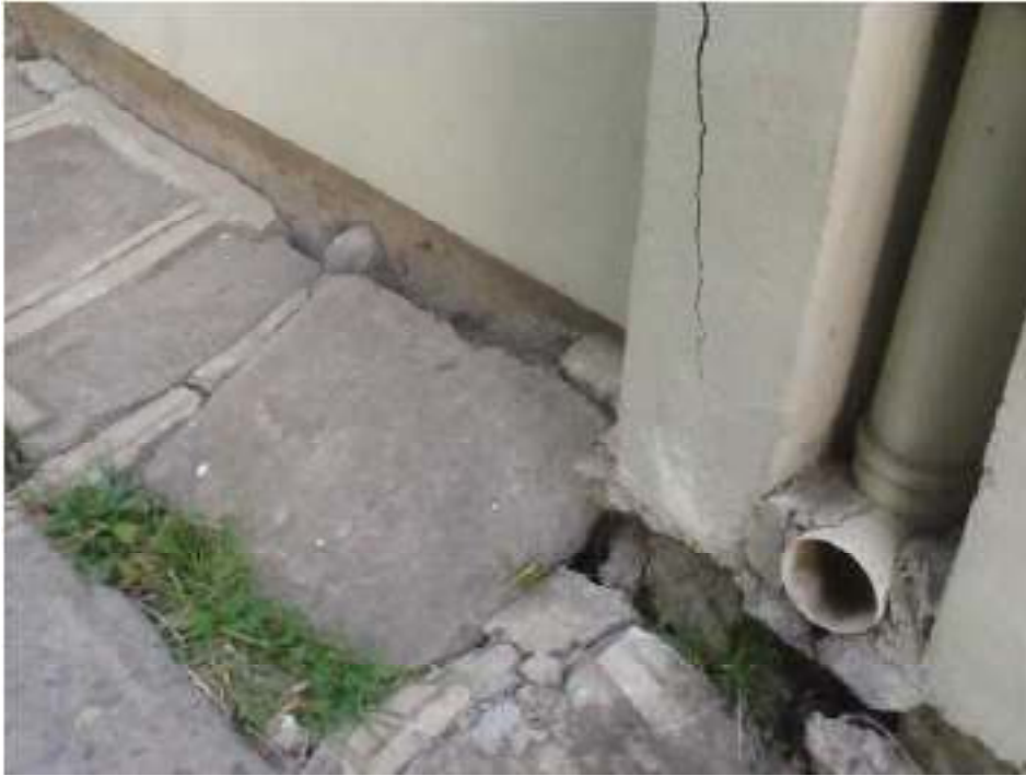
Figure 6. Separation of structure and walkway on Block 4
