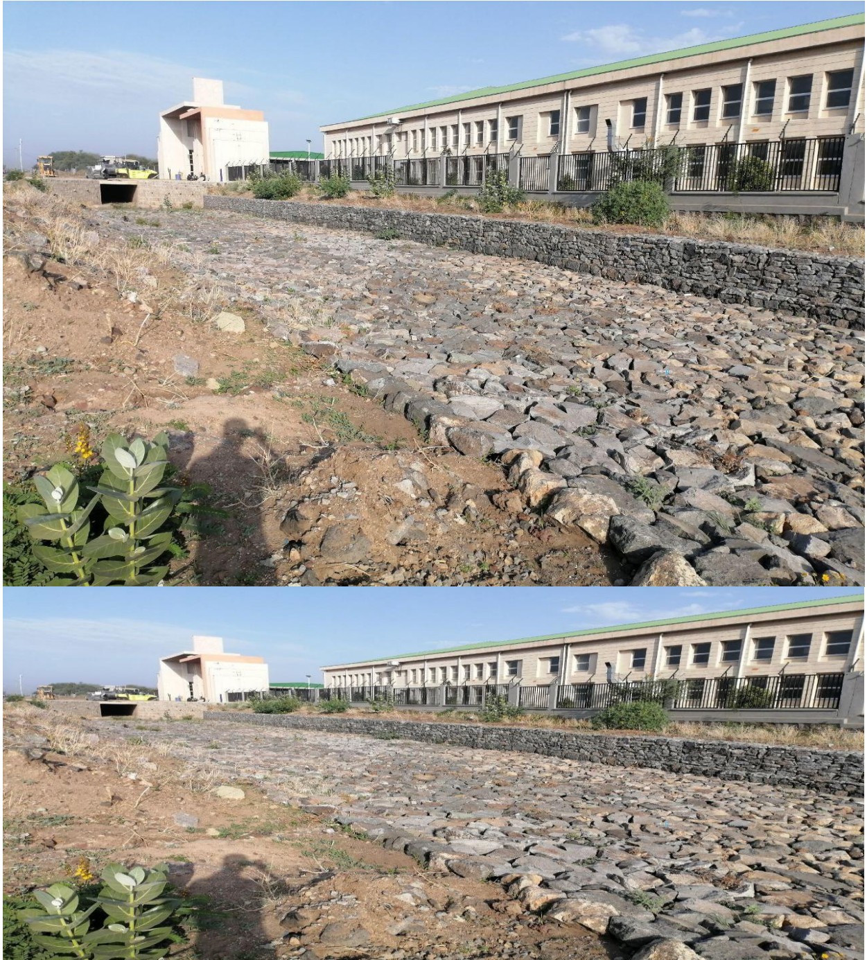
FIGURE 4.17: RIP RAP ARMOR AND GABION STRUCTURES CONSTRUCTED ON NATURAL STREAM CHANNEL AT OLENCHITI AGRO-INDUSTRY PARK FOR EROSION PROTECTION
