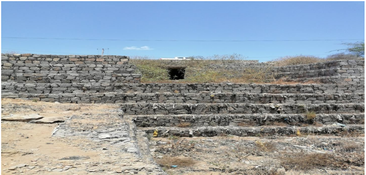
FIGURE 4.16: CONSTRUCTED GABION WALLS ON ETHIO-DJIBOUTI HIGHWAY AS EROSION PROTECTION MECHANISM
