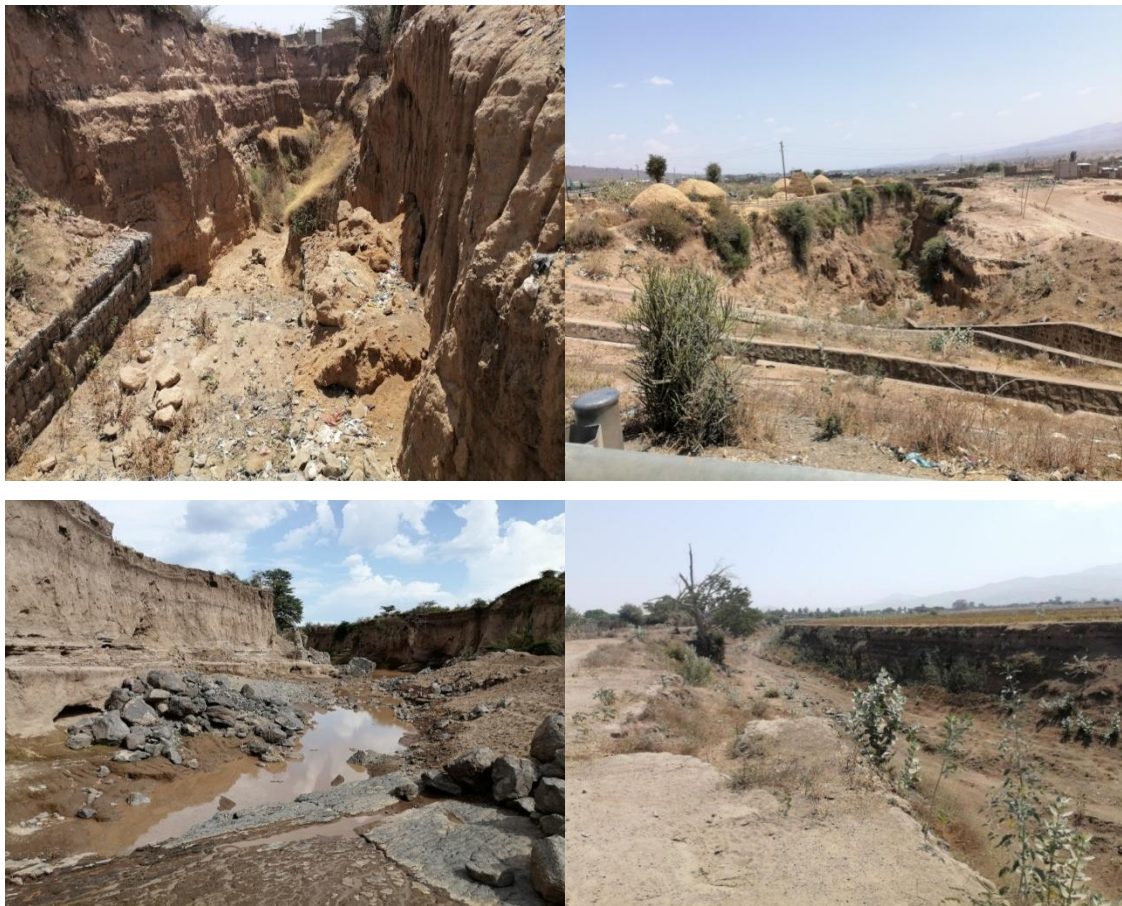
FIGURE 4.6: DEEP AND WIDE GULLIES FORMED BY EROSION ON THE STUDY AREA
