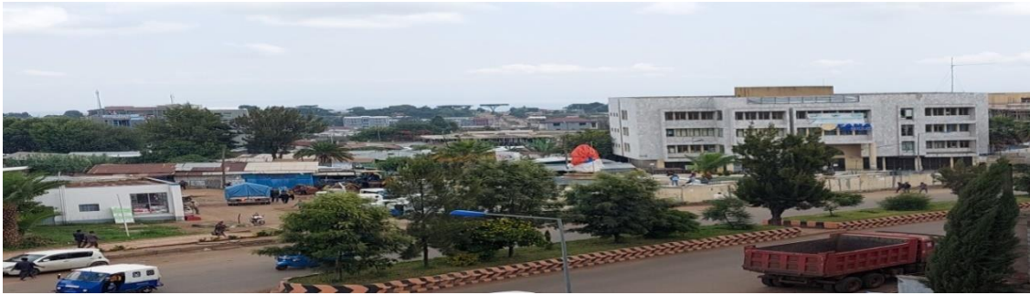
Figure 9: surrounding views of the building from terrace
