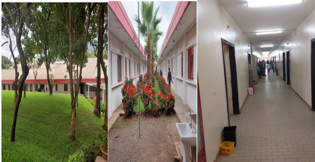
Figure 13: Construction material of the building and Artificial illumination
