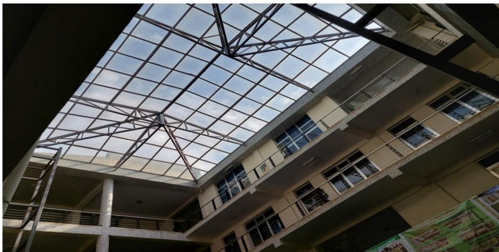
Figure 3: Open down and skylight of the building
