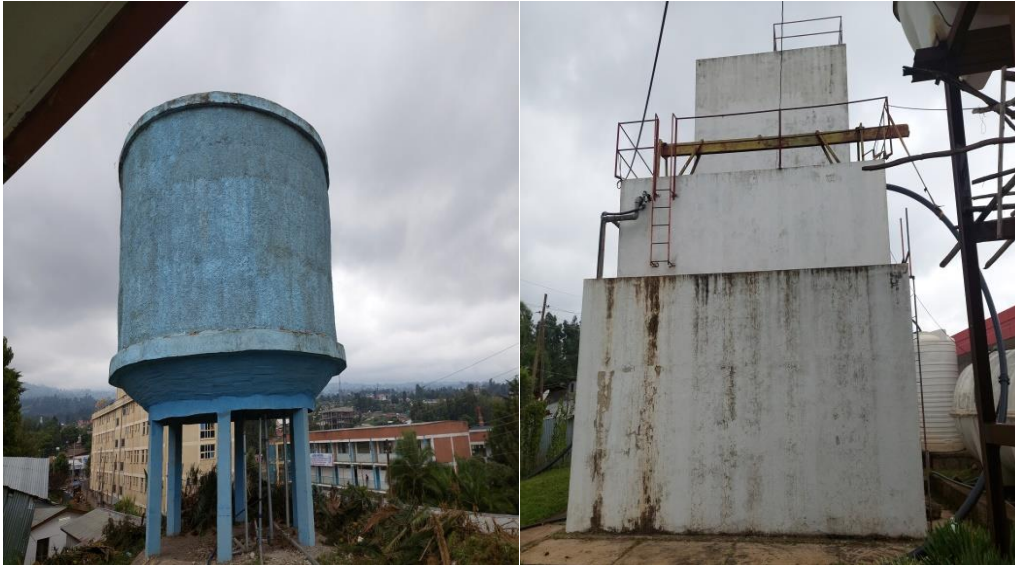
Figure 12: Water tanker of the hospital
