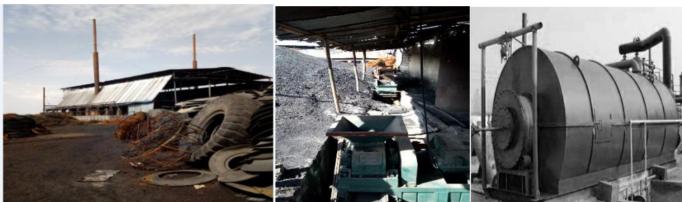
Fig. 15: Hang Wa pyrolysis plant
