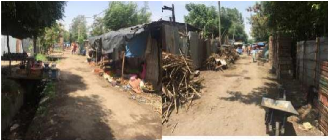
Figure 37 Shows Poor Quality of Roads in terms of Surface Material
