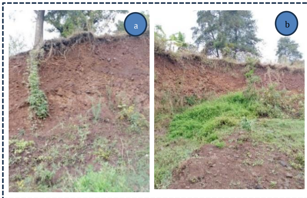
Figure 4. 6: Colluvial soil observed in the study area
