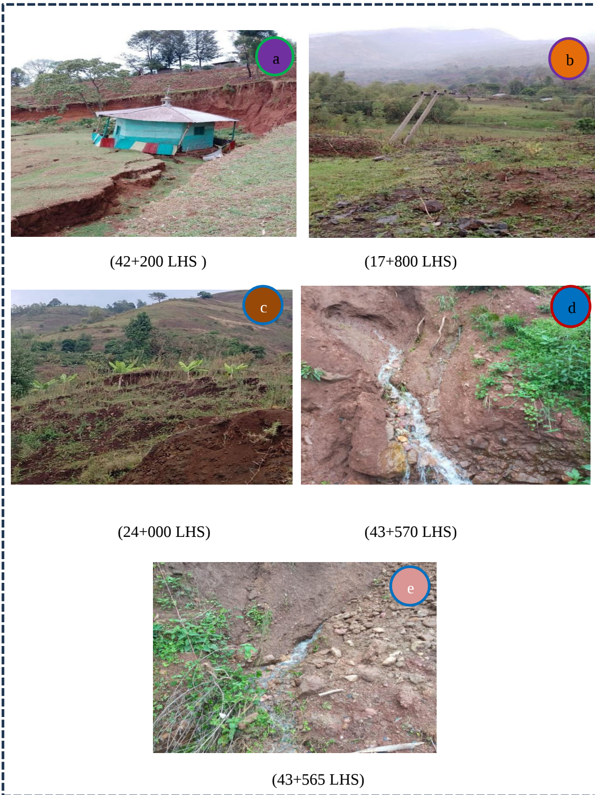
Figure 3. 1 a) Damaged church b) Tilt electric pole c) Damaged agricultural land (d) and (e) Springs observed
