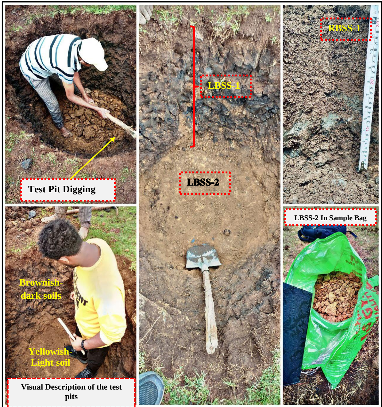
Figure 3.1. Test pit digging process and soil sampling from the test pit (LBSS-1, LBSS-2, and RBSS-1).
