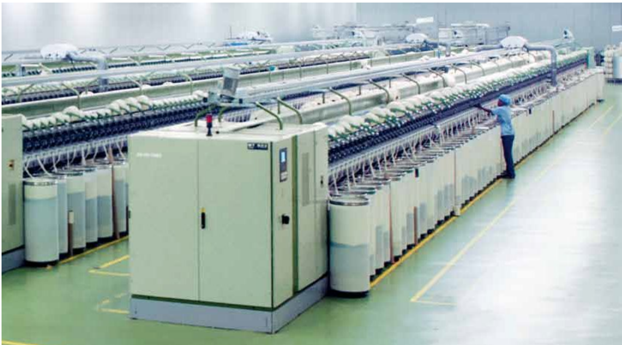
Figure 3.2: Adama Spinning Factory: partial interior view of the spinning plant.
