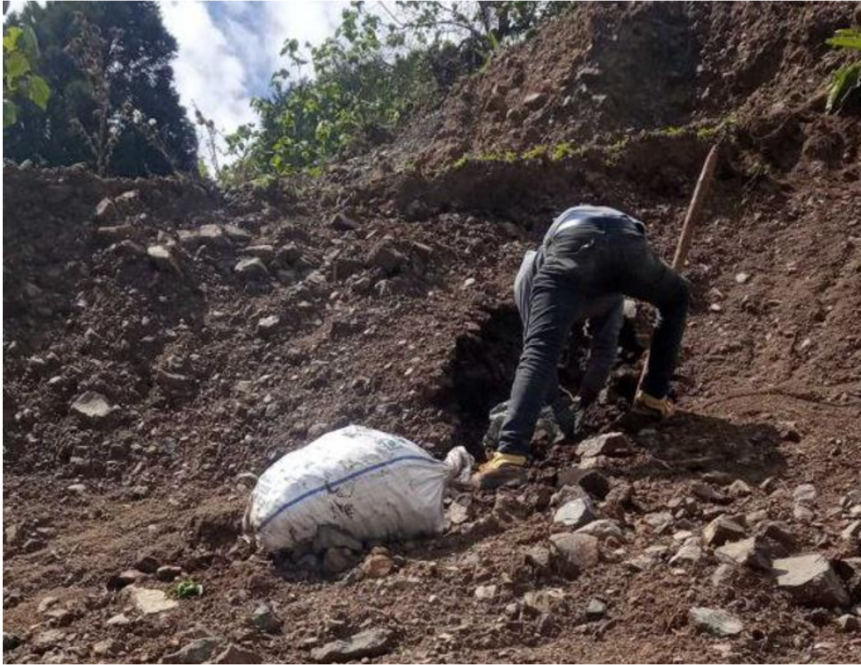
Figure 3-9 Pit Excavation sample taking at 12+078 for Laboratory Tests.
