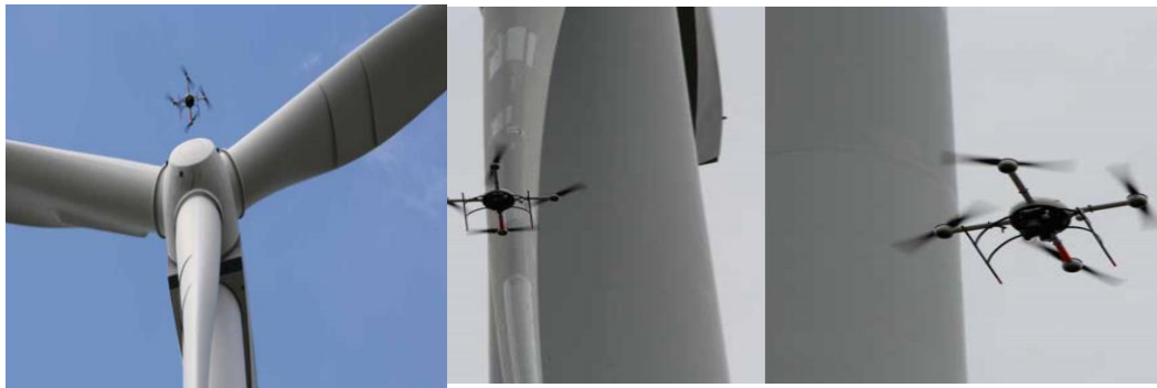
Figure 2.2 quad rotor for wind turbine inspection(Drone Inspection Guide Benefits & Industries Served, n.d.)
