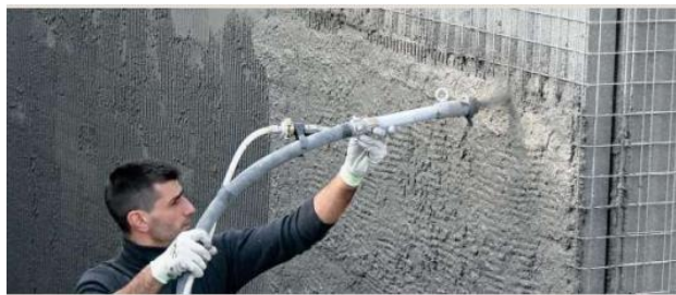
FIGURE 2. 7 Shotcreting of EPS Panel (Homes, 2018)
