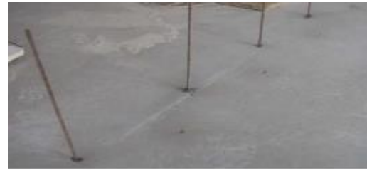
b) Drilled holes in the foundation Drilled holes in the foundation
