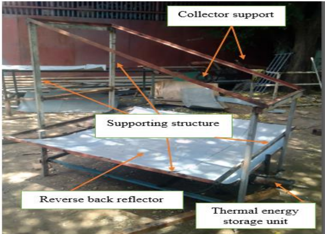
Figure 5. 6 Construction of Supporter Structure
