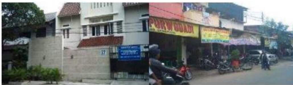
Figure 2.2 Street frontage at Grogol. Residential street (left), commercial street (right)
