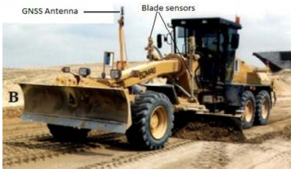
Fig.2. 6 Grader operation by automatic blade control system
