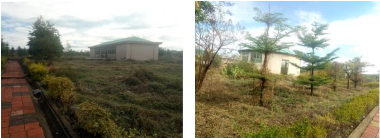
Figure 4.10: Site picture of the Current Condition of the Obo park
