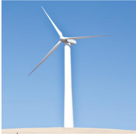
Figure 2.2 A wind turbine with a horizontal axis and three blades. (Burton et al., 2011)
