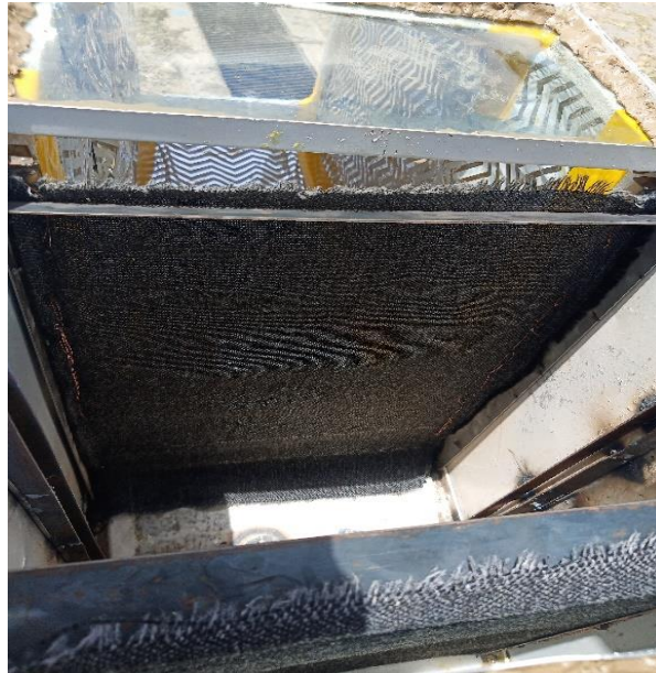
Figure 5. 5: Cooling pad
