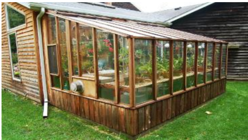
Figure: 2.7. Wooden framed greenhouses. https://sturdi-built.com/greenhouse-styles-sizes/greenhouse-kits-garden-sunroom/
