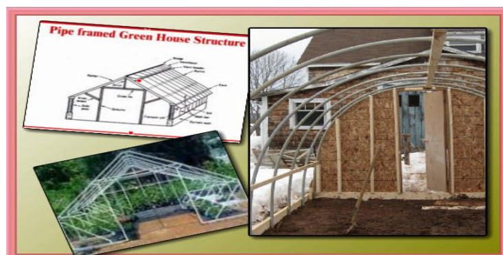
Figure: 2.8. Pipe framed greenhouse structures.
