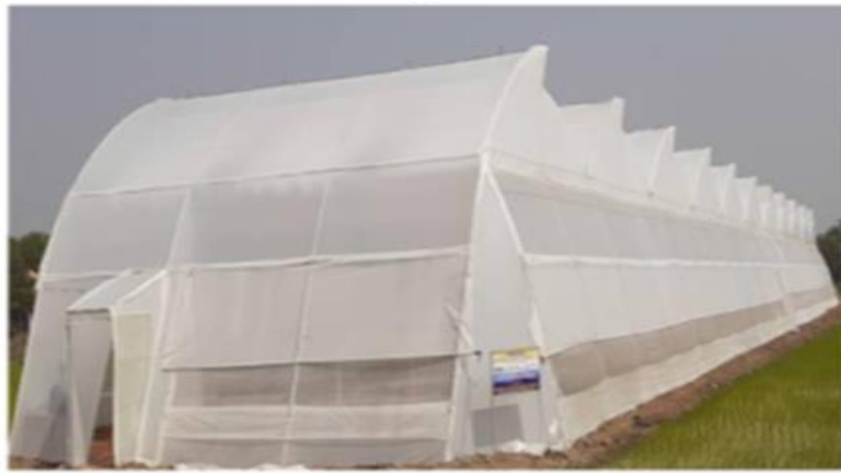
Figure: 2.5. Greenhouse with Sawtooth.
