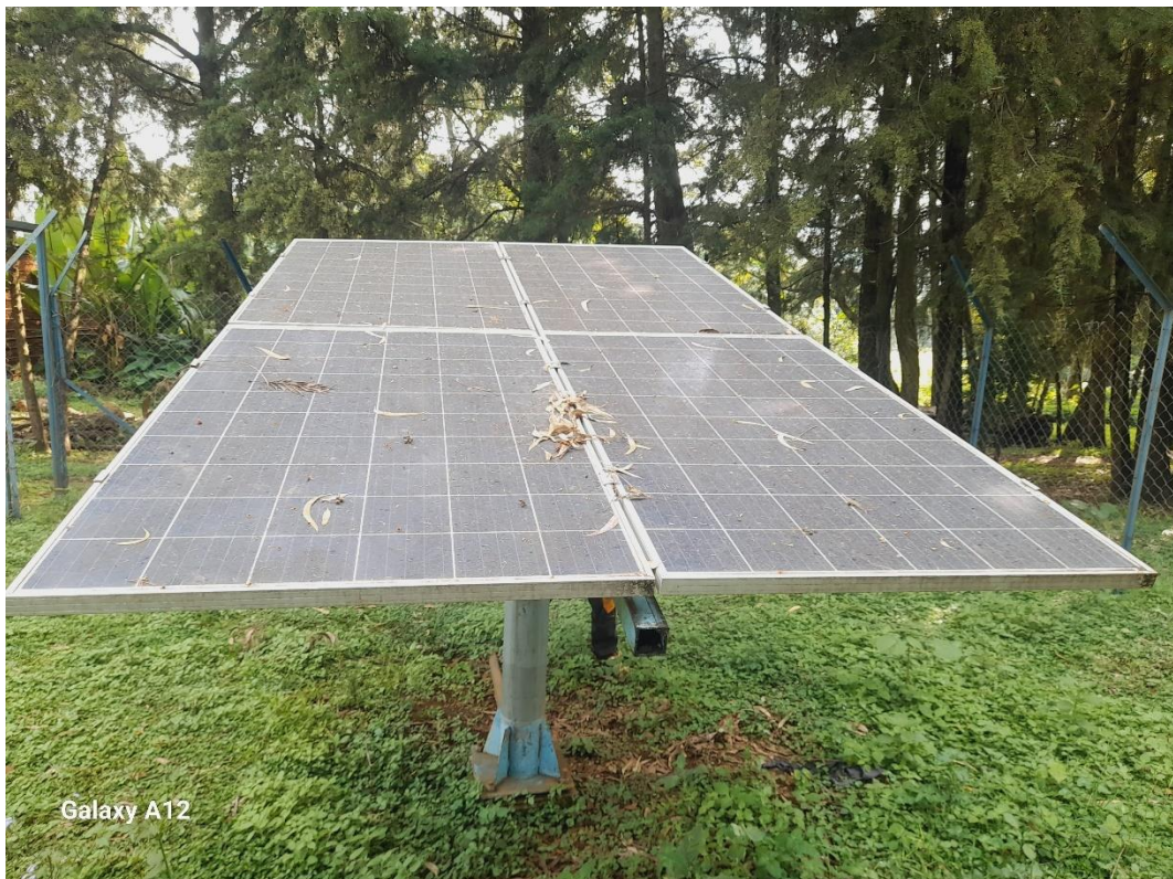
Appendix 15. A solar panel full of dirt in Dijala Village, Wormuma Kebele
