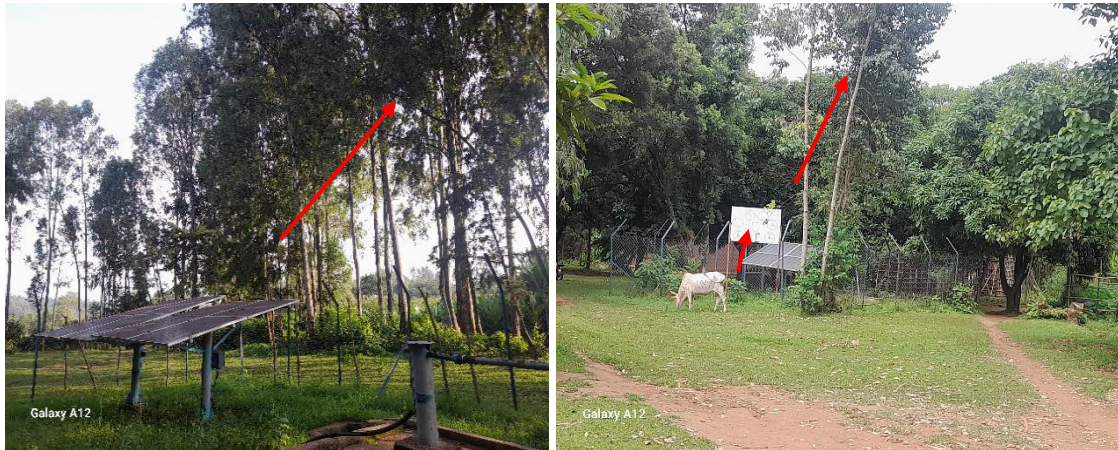
Appendix 14. Solar panels shaded under long trees in Dubo and Achura Kebeles
