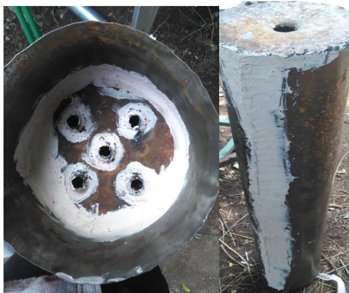
Fig 6.10 Filling the leakage opening using polyester putty
