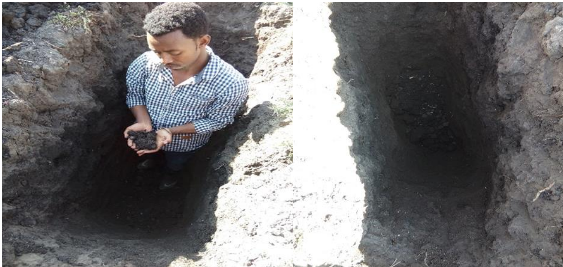
Fig C-6: when excavating for taking soil sample
