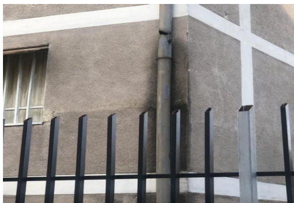
Figure 7-4 Broken downpipe
