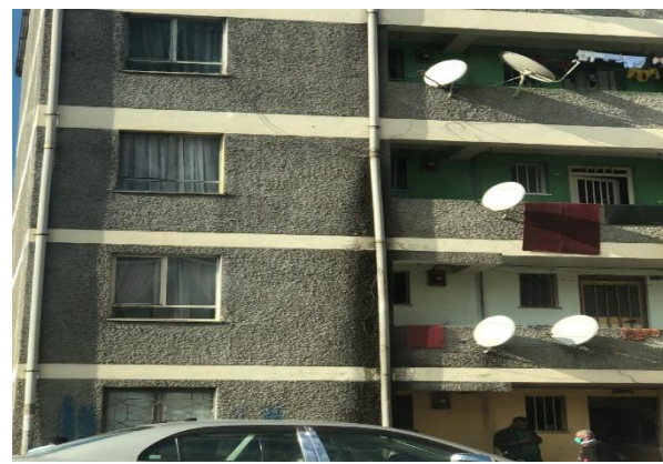
Figure 7-3 Broken downpipe
