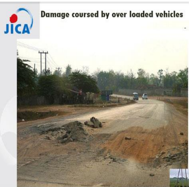
Figure 1. Pot holes developed because of heavy vehicles overloaded.
