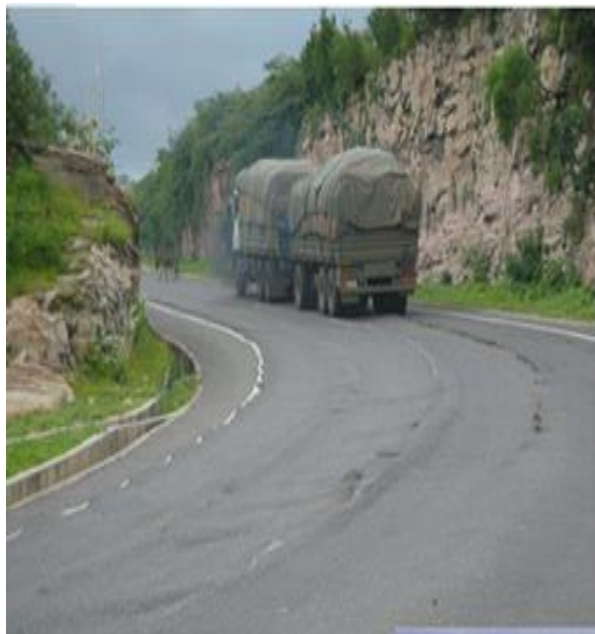
Figure 1. Pot holes developed because of heavy vehicles overloaded.
