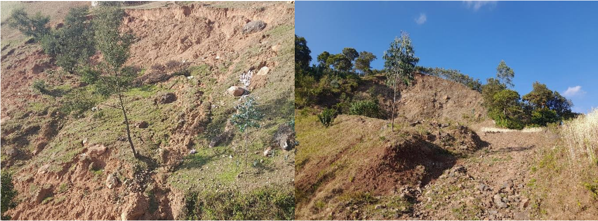
Debris slide landslide type
