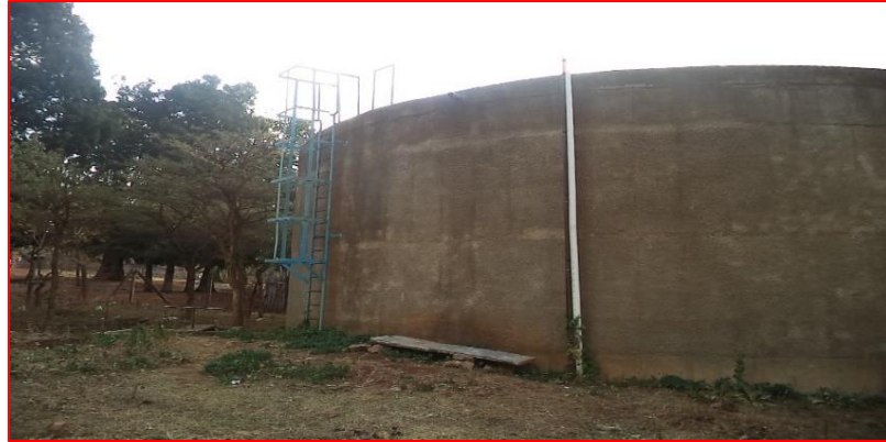
APPENDIX F: Gebriel reservoir located in kebele-12
