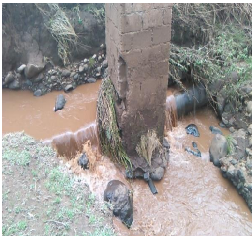
APPENDIX J: Exposed and damaged double orifice air valve in Mero dengego zone
