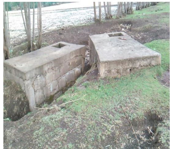
APPENDIX J: Exposed and damaged double orifice air valve in Mero dengego zone
