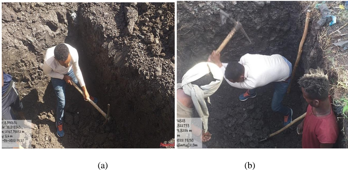
Figure 3. 2 (a) and (b)Photo of soil samples from Test pit one and Test pit two
