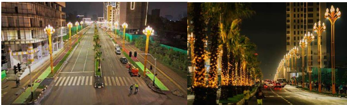
Figure 4.22: overall status of the street during the site survey
