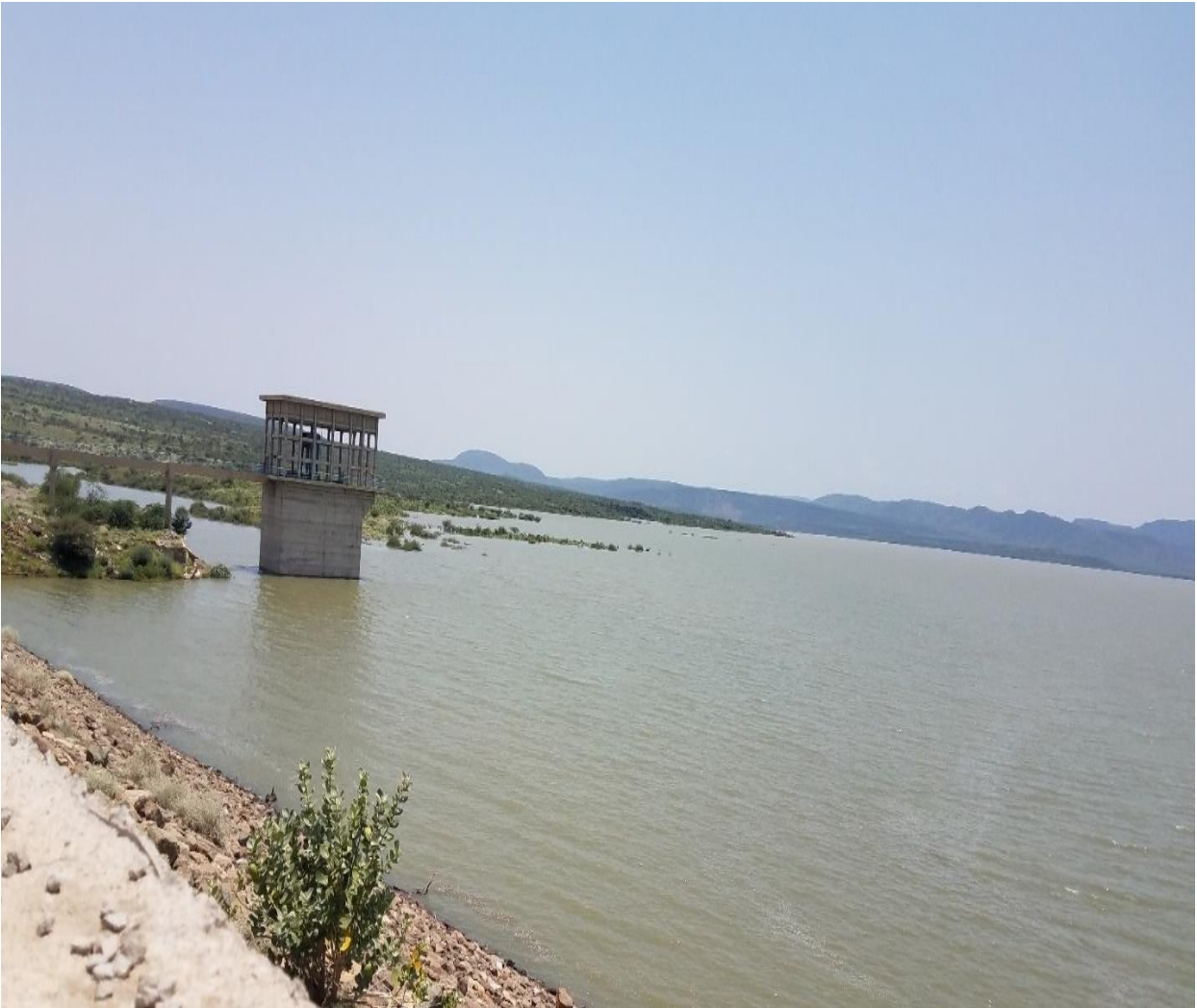
Figure 2.20: Kesem Kebena Dam
