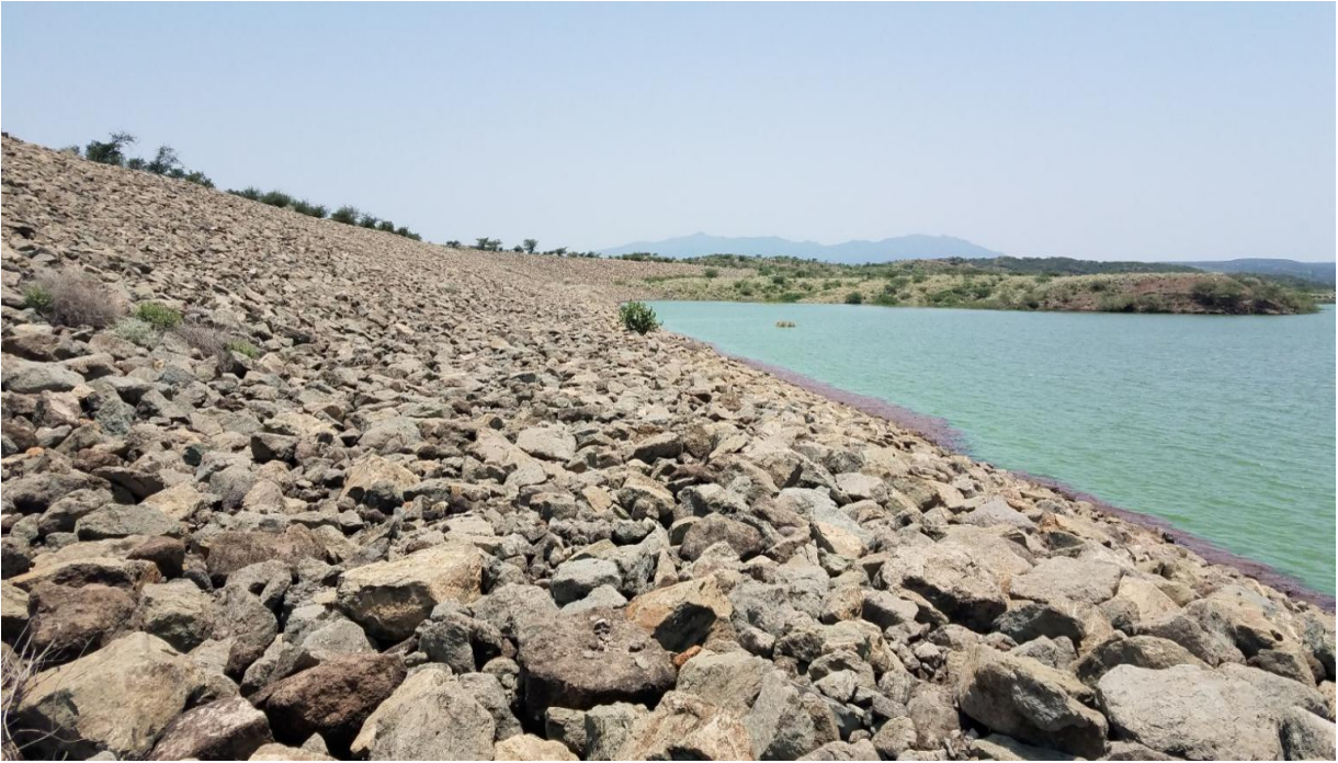
Figure 2.21 Kesem Kebena Dam
