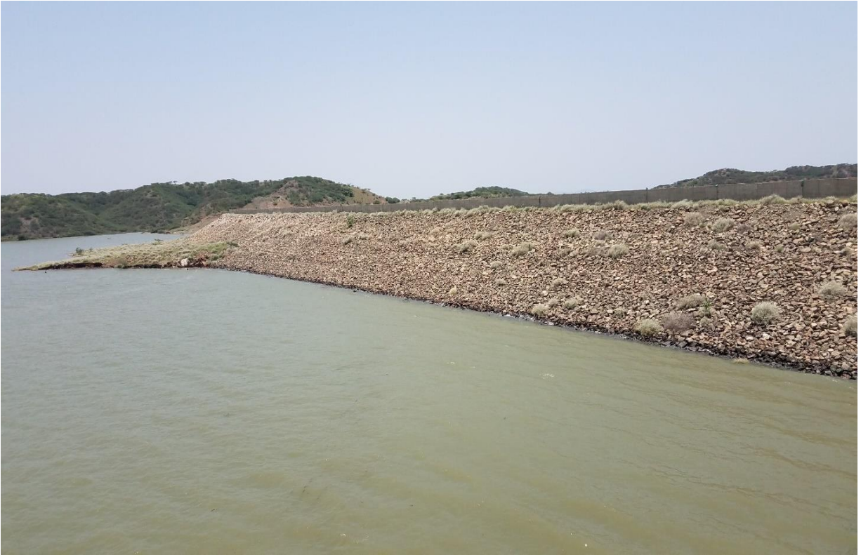
Figure 2.23 Kesem Kebena Dam structure view
