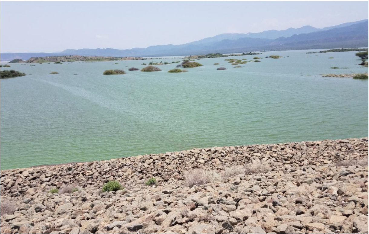
Figure 2.22 Kesem Kebena Dam water level view
